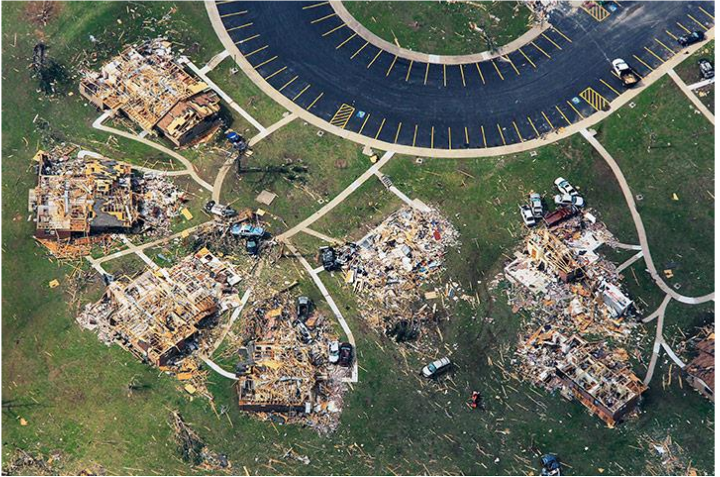
An aerial view of destroyed houses in Joplin
